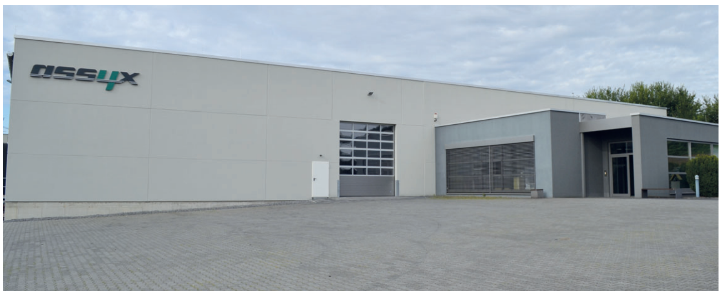
A second hall aisle was added to the existing production hall.
